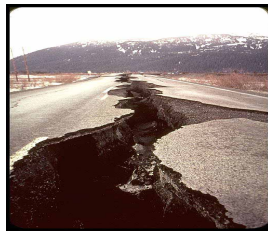
14 Cracks in the street after earthquake
