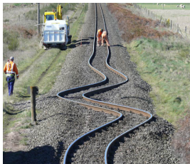
13 Distorted railway line after Canterbury earthquake, New Zealand, 2010
